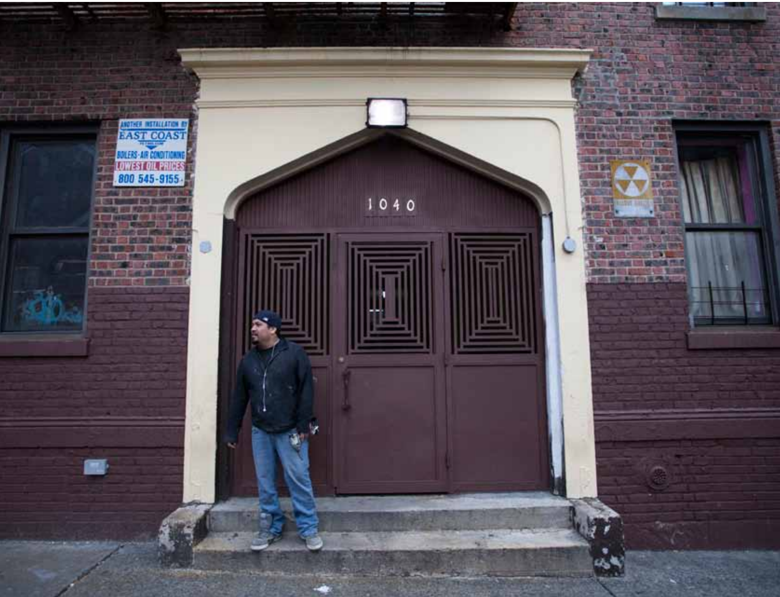
1040 Boynton Avenue, a building owned until recently by companies linked to Frank Palazzolo, sported 210 housing code violations at press time. Photo by Marc Fader.
